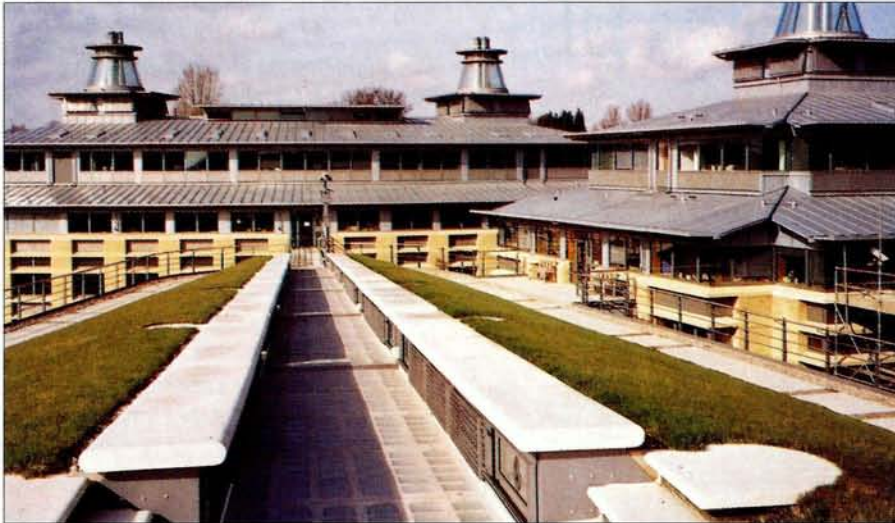
Striking architecture at Cambridge University's new Centre for Mathematical Sciences. The Cambridge mathematics department has a proud tradition in theoretical physics, encompassing the work of Newton, Dirac and Hawking. Today some 100 staff and research students work in particle physics and cosmology. Faculty members have been raising funds for new buildings on a site that they will share with the Isaac Newton Institute for Mathematical Sciences and a major new science library. The theoretical physics building is named after Måril and Hans Rausing, Swedish-born Rausing was the managing director (and later chairman) of the Tetra Laval Group for almost 37 years. The library is named after Betty and Gordon Moore. Moore, a co-founder of Intel, invented Moore's law, which predicted the growth of computing power. This picture shows the development of the half-completed centre. Construction of the remaining buildings is just starting. In two years the faculty and the library will have nearly 20 000 m 2 of space. For more information see " http://www.cms.cam.ac.uk ".
